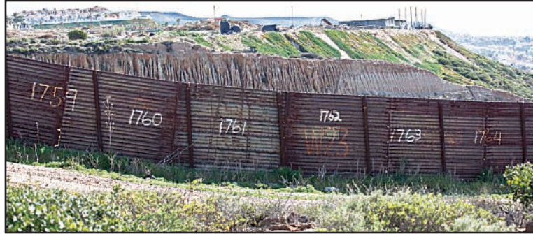
Photo above: an already existing border fence near San Diego. More than 30 laws were waived to begin additional border wall construction near the city.
