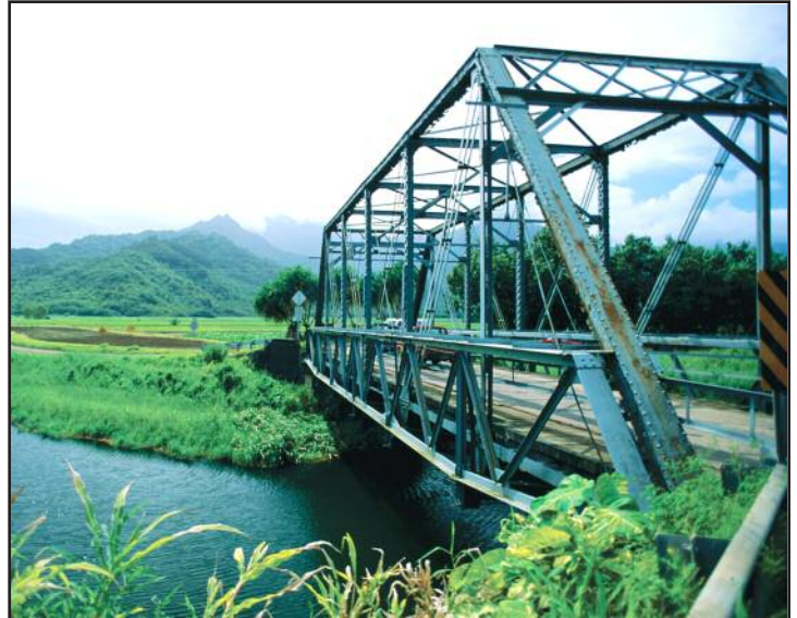
The one-lane bridge to Hanalei, Kauai, with its 15-ton capacity, helps keep big development out.
