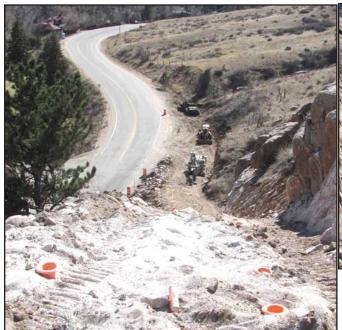
this is dangerous work any way you look at it. After the holes have been drilled, inverted orange construction cones were inserted to hold the soil back. The placement, depth, angle, and amount of charges are calculated by drilling and blasting experts and geologists, who quickly evaluate the blast results and make any necessary adjustments. Every blast in fractured rock face is a learning experience, and how the rock
