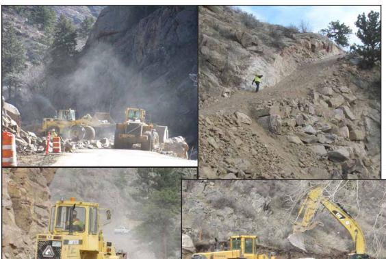
clear out my car. As one supervisor simply put, "They hustle." After the rock is cleared, some is pushed over to reinforce the river bank and some is transported out, a forklift fitted with a "broom," a rotating circular brush made of nylon, plastic and metal, is used to sweep remaining debris off the road until the striping and edge of the road are visible. After final determinations were made to remove the first 25' tier of the hillside near the pit, a few more holes were drilled to set the
